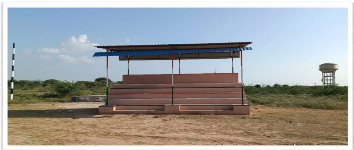
Construction of Pavilion work near our plant area, Khejarla
